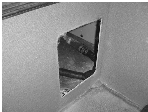
Figure 7 - Return air vent hole cut
