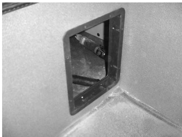
Figure 8 - Return air grill flange installed
